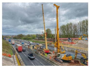
this scope of works was complete, there was further demobilisation and movement to the central pier, where piles were installed between the two 50mph running lanes of the M56. The final demobilisation and remobilisation was into the east abutment, to complete Bauer's scope of works.
