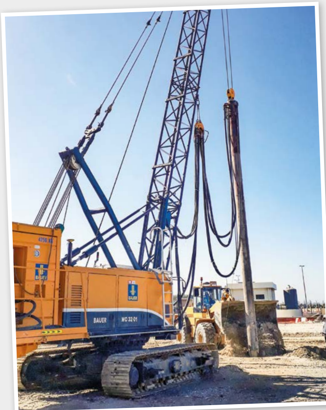
Completion stage, with the crater being filled with suitable material.
