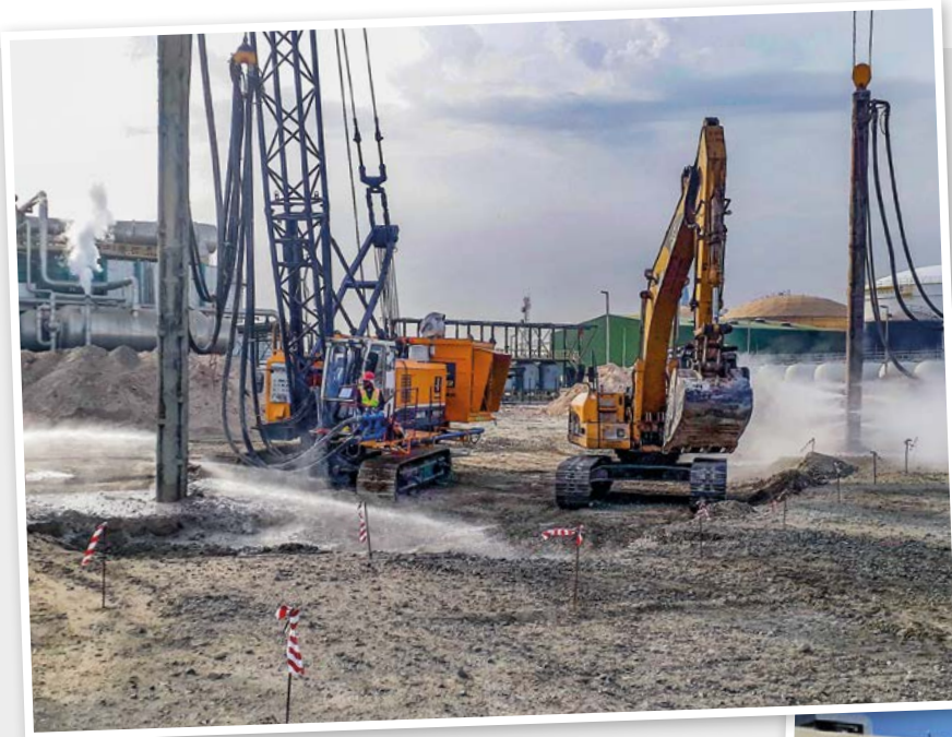
Compaction stage aided by air and water flushing.
