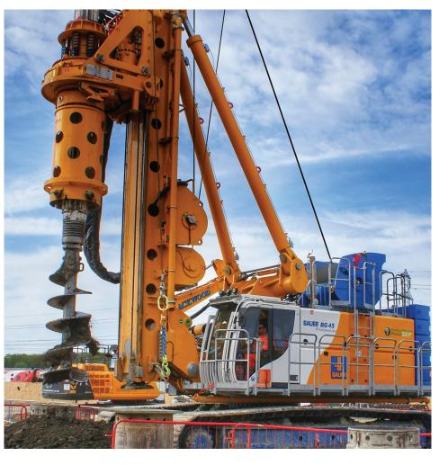
For example, the 183No piles required for the TBM Launch Pit (Phase I) was an increase on an original scope of 120No piles; the TBM Launch Pit was increased in length to aid later construction of a syphon for the Werrington Brook that passed through the site. Piling was also expected to be wet, however Bauer quickly discovered that the piles were dry and that the BG45 drilling rig had more than enough torque to drill the strong Cornbrash Limestone, which was encountered at 11m to 13m depth.
