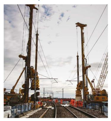
Bauer Technologies was awarded a £3.5m sub-contract by Ferrovial Lagan JV (FLJV) to install the foundation piles for a number of structures along the new motorway, including the 8no. 2.0m diameter foundation piles for the Braehead Railway Bridge.
