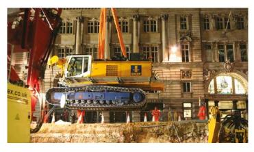
Bauer Technologies completed the Crossrail Advance Works Contract C501 at Moorgate, London in August 2013. The contract, for main contractor BAM Nuttall Kier Joint Venture, included extensive pile probing and removal, using the Bauer Technologies developed Annulus Cutter.
