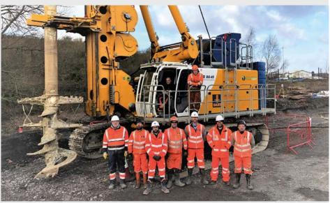
The ground improvement was installed by means of Ø2000mm Deep Soil Mixing (DSM) columns, to maximum design depth of 11.50m, using a BG45 piling rig and associated grout mixing plant.
