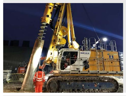
Bauer was appointed by tunnelling contractor, STRABAG International, to install a secant piled shaft, together with the bearing/ tension piles required for the overground shaft equipment.
