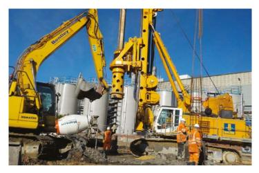
As the work was to be undertaken while the chemical plant was in operation, the project was not without its challenges. Specifically Bauer Technologies had to install a number of rotary bored piles in close proximity to BASF's existing chemical storage tanks, which carried inherent risk as well as influencing construction sequence.
