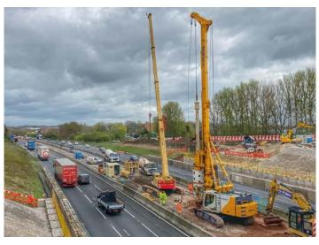
this scope of works was complete, there was further demobilisation and movement to the central pier, where piles were installed between the two 50mph running lanes of the M56. The final demobilisation and remobilisation was into the east abutment, to complete Bauer's scope of works.
