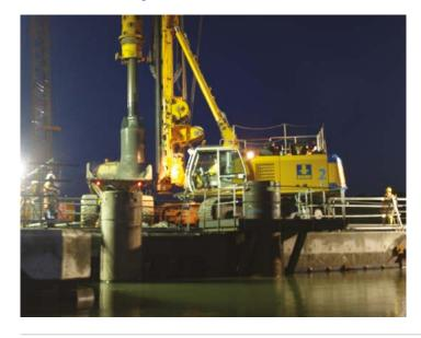
Bauer Technologies completed these extremely complex works on a 50 year old jetty on the Severn Estuary at the site of the new 2000MW, Combined Cycle Gas Turbine Power Station, to support the Leibherr LGD 1750 crane and its 387.5 tonne superlift required for the safe off-loading of five 400-tonne gas turbines as part of the stations' construction.
