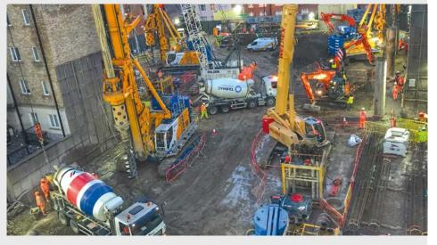
Obstruction coring and old pile removal was also performed, as some pile locations were obstructed with in-ground features, including existing slabs, old piles, and concrete thrust blocks.
